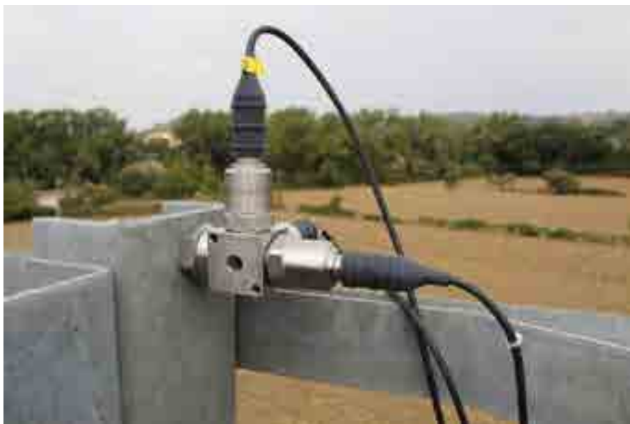
Figure 79. Accelerometer mount on the top part of the guardrail.
