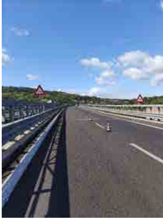
Figure 66. View of the road from on top of the deck.
