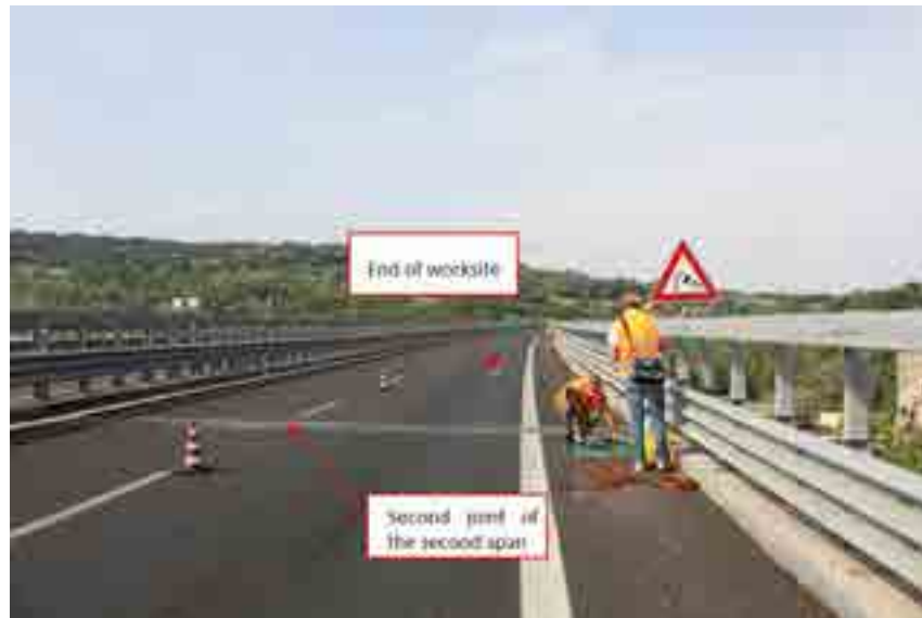
Figure 76. Third view of the worksite.
