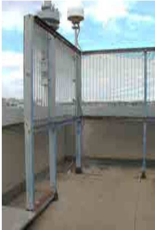
Figure 11. West-North corner of the SOGEI structure.
