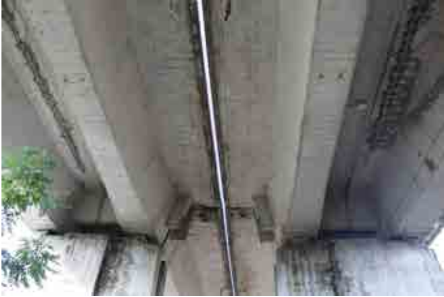
Figure 68. Details of the four box girders.
