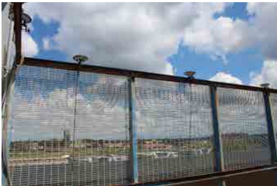
Figure 32. Fourth view of the GNSS system configuration.
