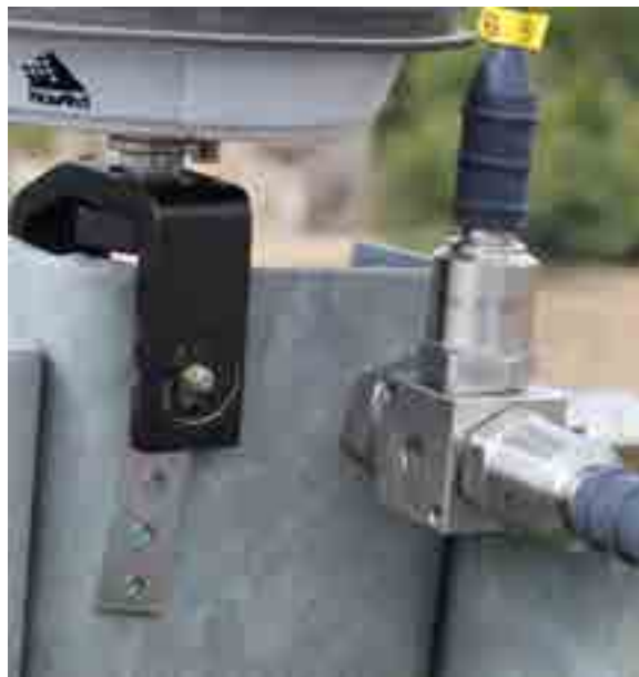
Figure 25. Installation of the NovAtel antenna and the accelerometer.
