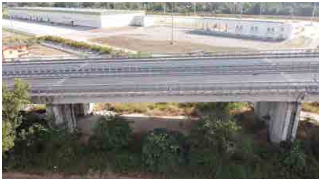
Figure 65. Drone view of the second span of the bridge.
