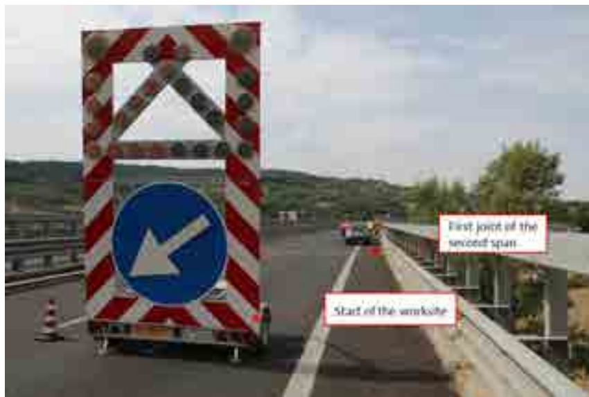
Figure 74. First view of the worksite.
