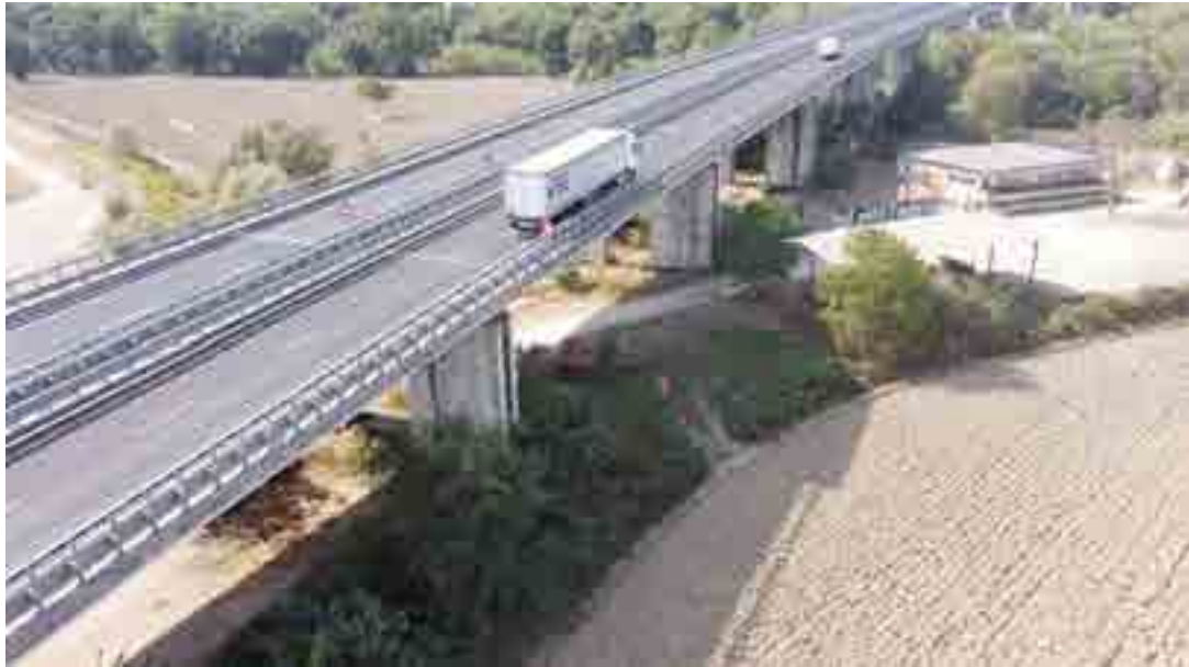
Figure 64. Drone view of the road bridge.
