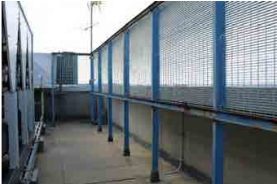
Figure 10. West-South side of the SOGEI structure.
