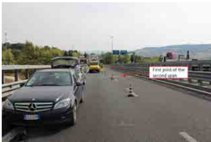
Figure 75. Second view of the worksite.
