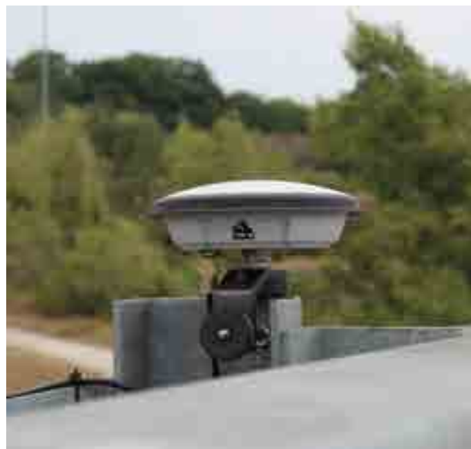
Figure 77. Antenna installed on guardrail.
