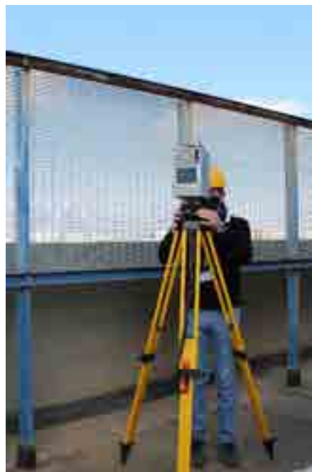
Figure 13. Surveying with laser scanner technique.
