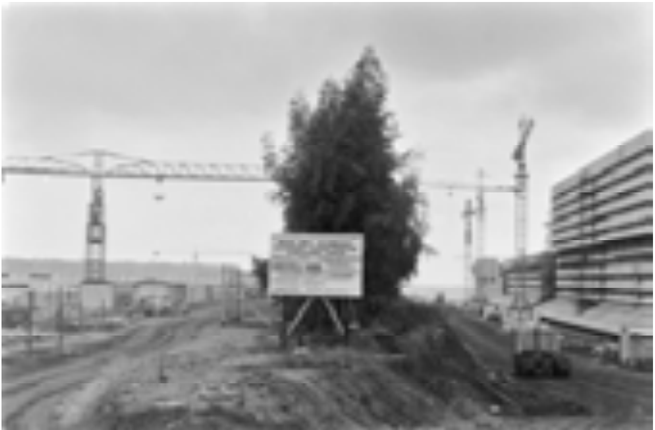
Figure 4. Corviale construction site. Photo: Aldo Feroce.
